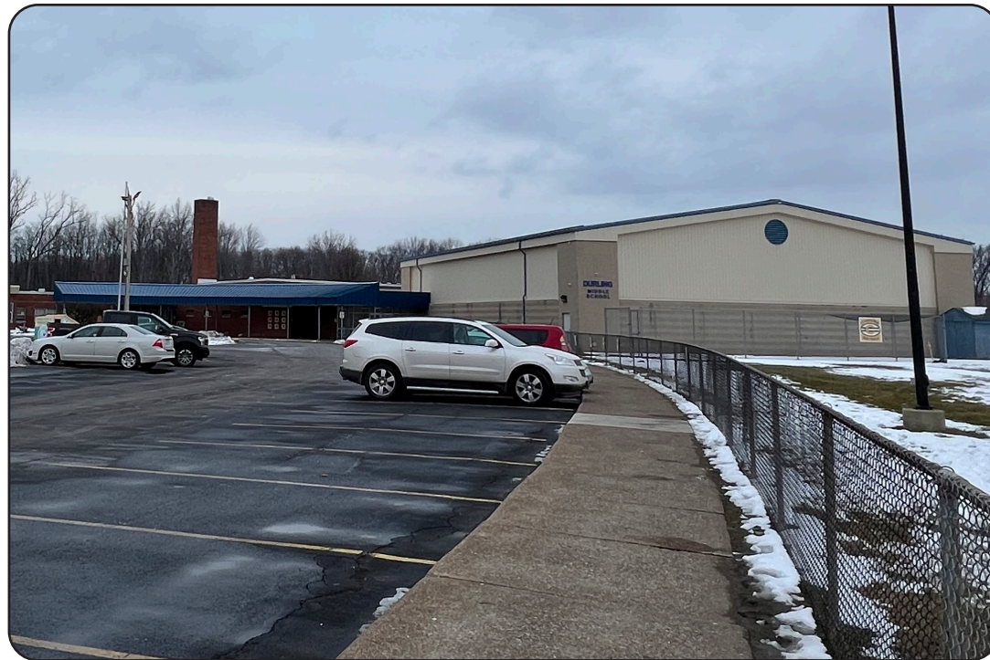
The Durling Middle School building from the parking lot.
